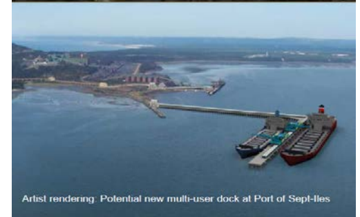
Dredging commenced for new multi-user deep water dock
