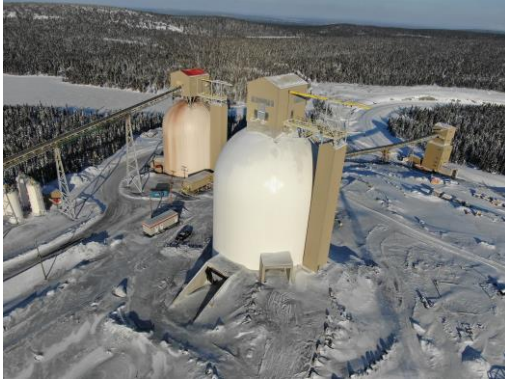
Reclaim conveyor structure assembly ongoing
