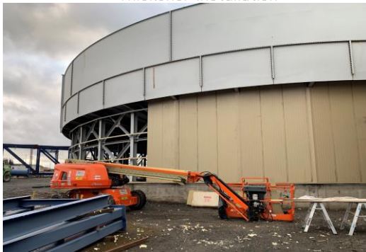
Thickener installation
