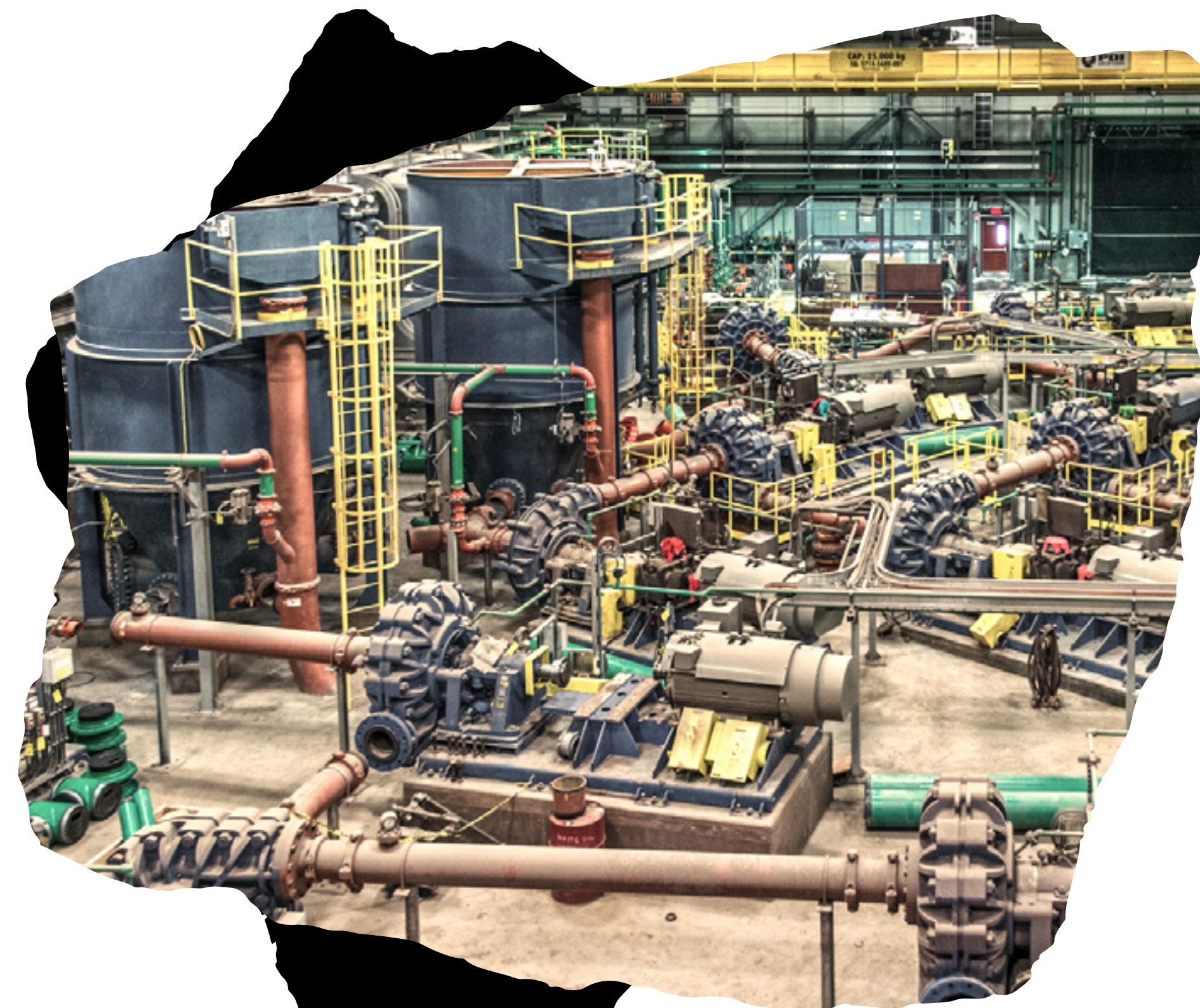
Booster station used to pump tailings
