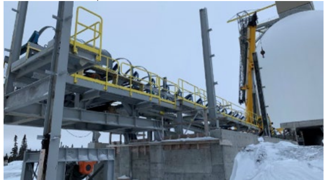
Load-out – Conveyor 6 structure erection
