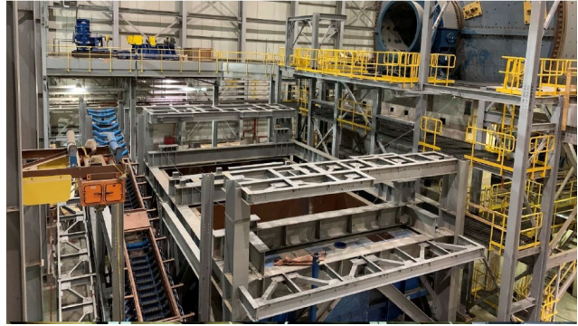
Load-out – Conveyor 6 structure erection
