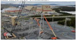
Structure steel work in the milling and screening area
