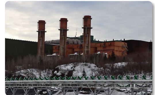
Pointe Noire Pelletizing Facility
