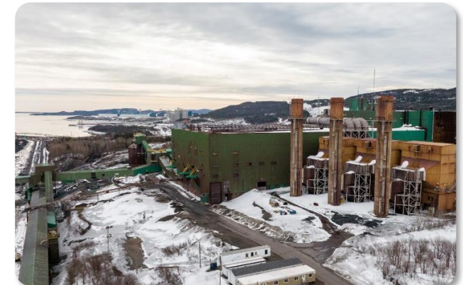
Pointe Noire Pelletizing Facility
