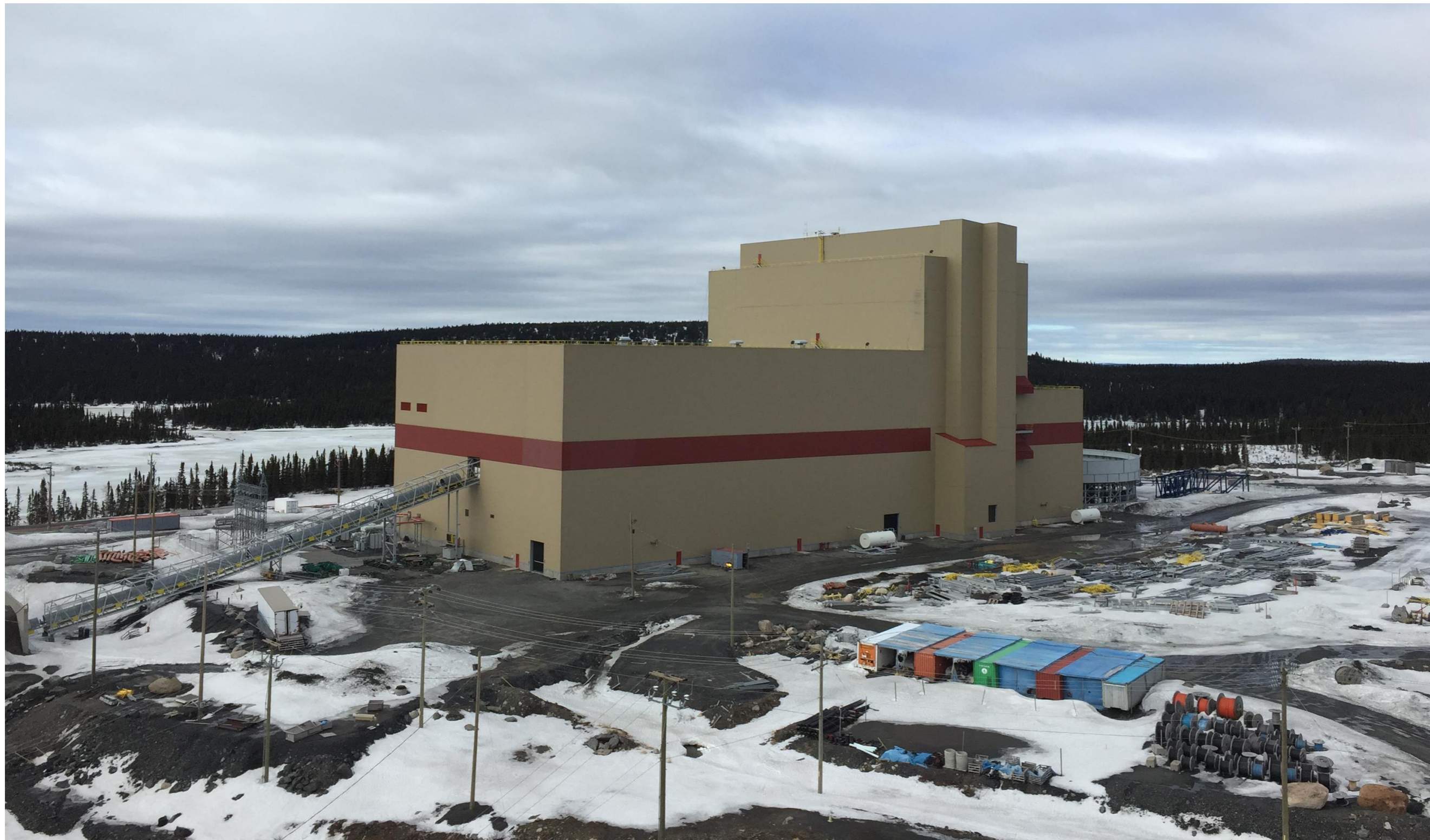
Figure 18-2: Constructed Phase 2 process plant
