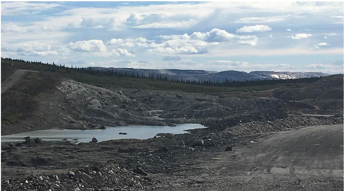
Figure 15-2: West Pit overburden striping
