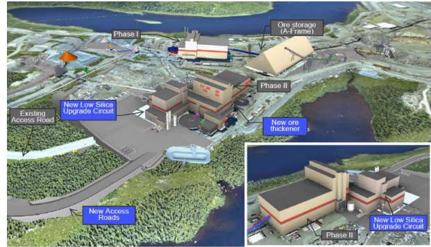
Source: Champion Iron Limited; Rendering of the Phase II concentrator including the proposed modifications for the DRPF project
