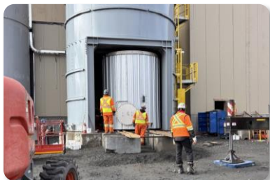
Exterior work – South
